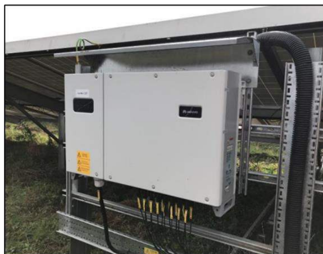
Figure 2-1: Typical String Inverter
